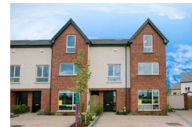
Bellingsmore Housing Development
